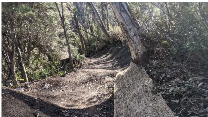
Figure 5. Example shows the trail following the contour of the slope, rather than down the fall line
