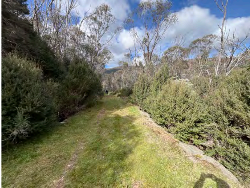
Figure 15: Trail follows the existing disturbed ski run and access corridor and utilises its existing culverts
